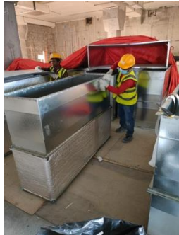
Duct Insulation Installation
