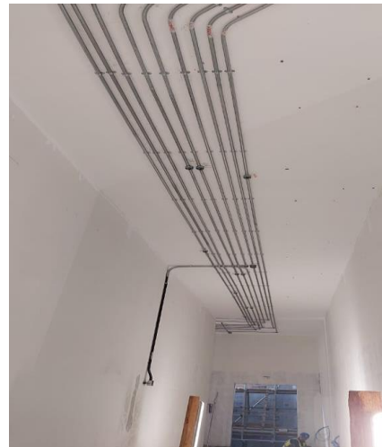
Lighting Pipe installation
