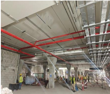
Fire Pipe Installation
