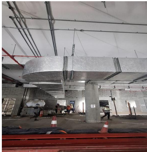
Duct Insulation Installation
